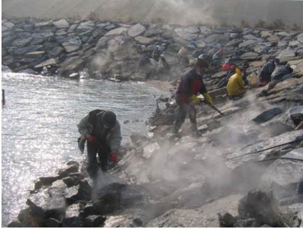
Contractors used hot water high pressure treatment at some sites
