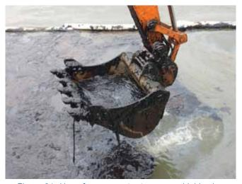
Figure 21: Use of an excavator to recover highly viscous fuel oil. The concentration of recovered oil was maximised by instructing the operator to hold the bucket above the water surface for a short period, to allow entrained water to run off. This reduced the subsequent disposal costs at the expense of recovery efficiency.
