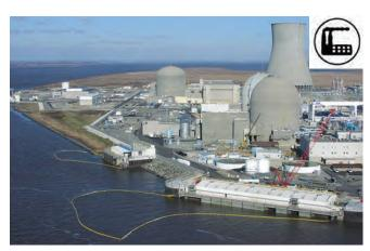
Figure 6: Power station with a water intake in the foreground. Several deflection booms are deployed to prevent the ingress of oil.
