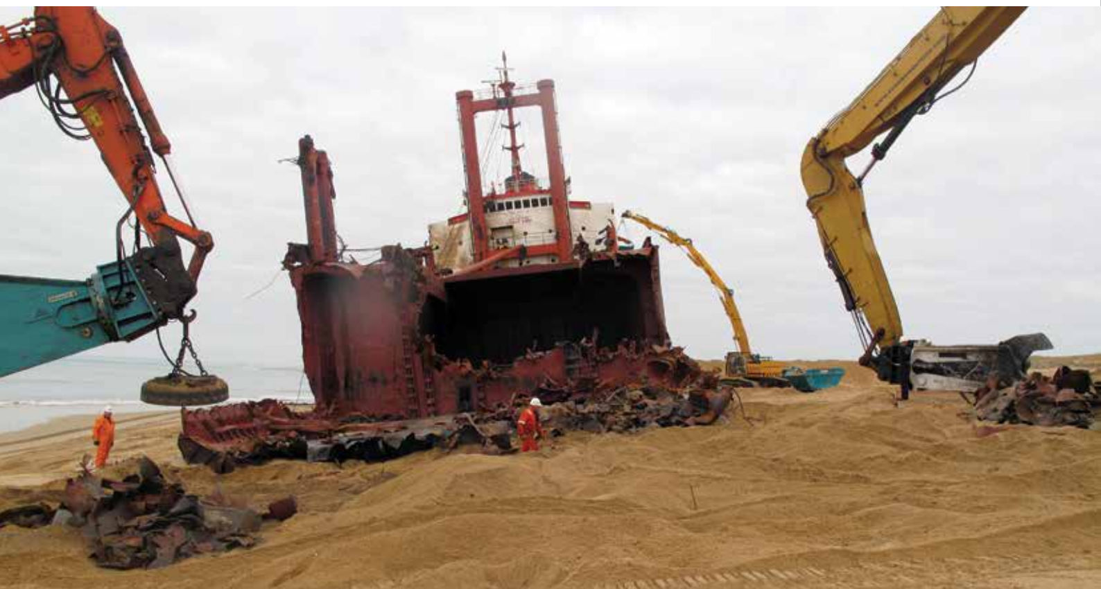
▼ TK BREMEN being demolished on site
