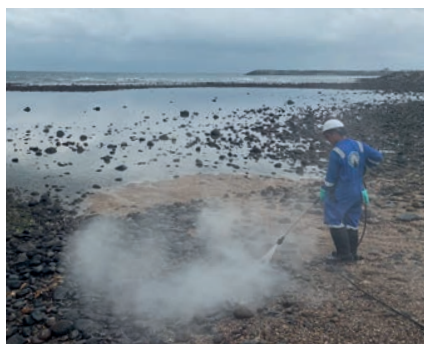
Pressure washing cobbled shoreline, UAE
