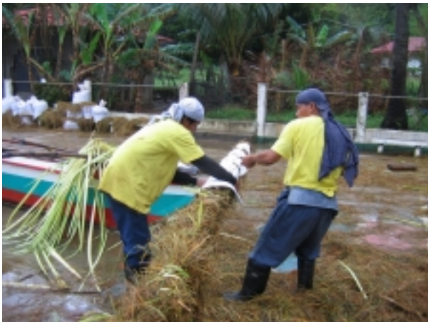
Artisan booms using bamboo and grasses were deployed at several sites in an effort to protect coastal resources.
