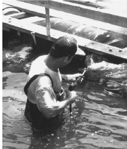
Figure 1. Cleaning of mariculture structures can be difficult and time consuming.
