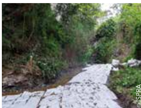
Protection of a working area with sorbent sheets
