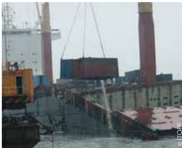
Recovery of collapsed containers
