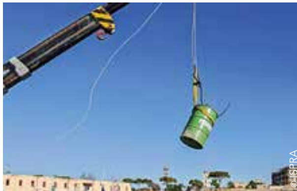
Lifting a drum with a crane
